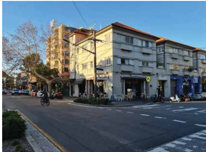
Terracotta-tiled roof building, unifies the North & South of the site.
