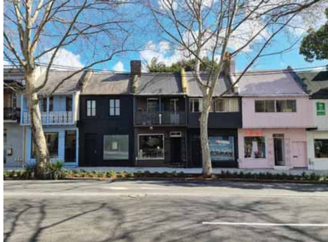
Terraces along South Downling Street, mainly retail and commercial
