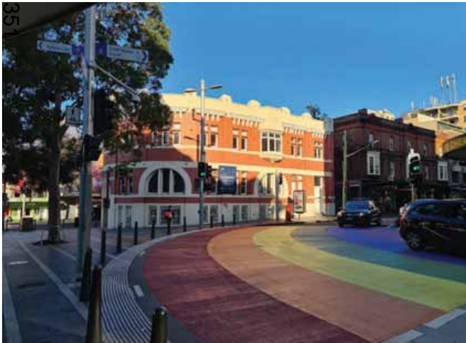
Rainbow crossing enhances visual appeal of the block The simplicity of the creative endeavour from the coloured pavement far outweighs the visual appeal generated by Taylor Square itself.
