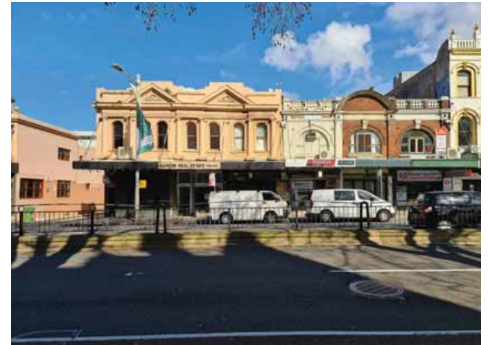
Victorian terraces with potential to be heritage listed.
