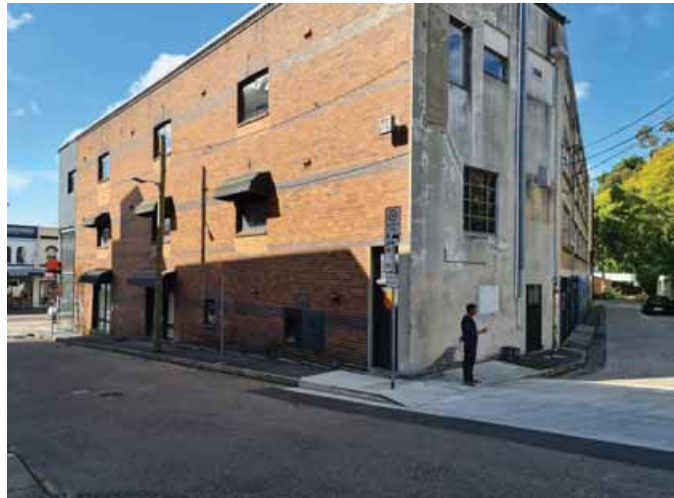
Inactive facades on Verona Street, older layers don't mix with new addition
