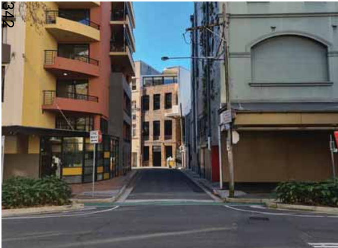
Limited accessibility to Little Oxford Street
