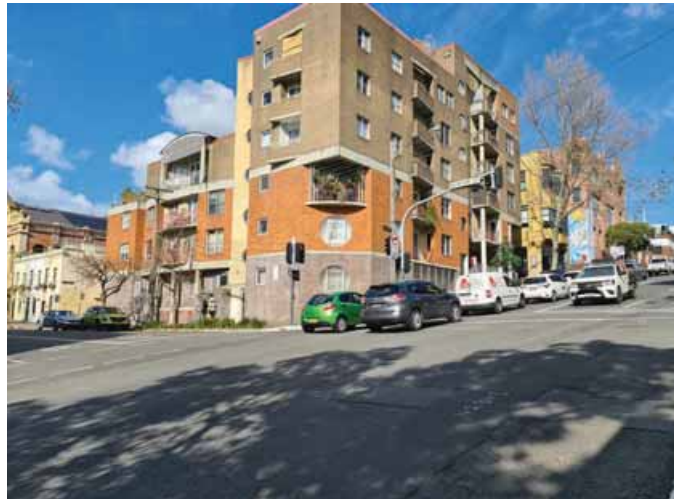
Social Housing building at 254 Crown Street
